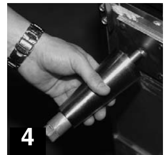
4 Thread leg into cabinet bottom frame rail.
